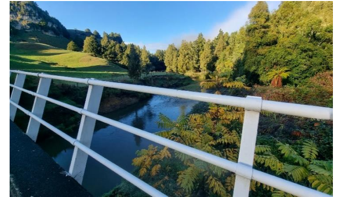
The Mangaotaki Bridge
